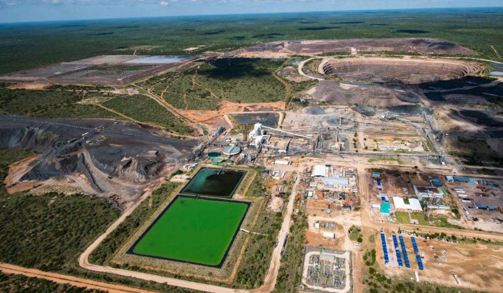
Aerial view looking west displaying water storage, processing plant and open pit
