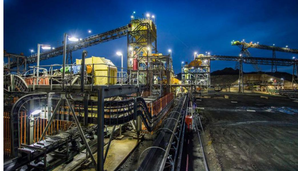
Karowe processing facility and tertiary crusher building
