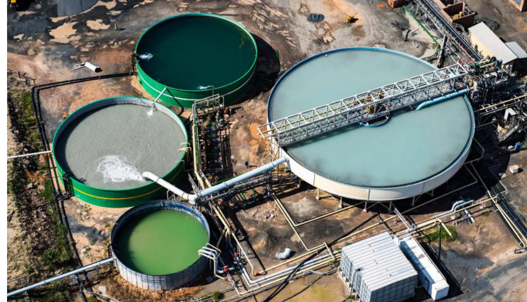
Thickener and processing water storage
